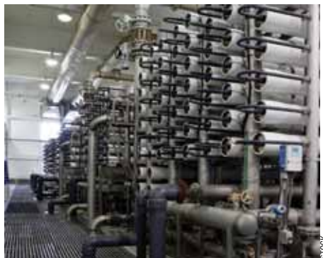
A reverse osmosis system, such as the one shown here, is used in a sewage treatment plant to filter inorganic salts that remain in the water.
