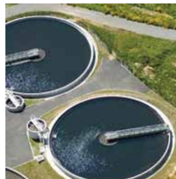
Aerial view of settling tanks at a sewage treatment plant. Large pieces of materials settle at the bottom of these tanks and are later removed and reprocessed.
